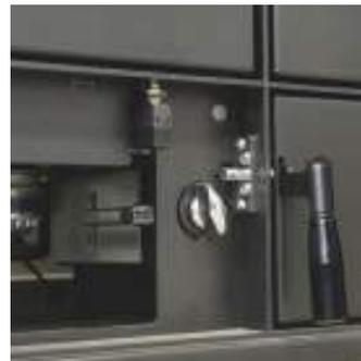
**THERMOSTAATKLEP VOOR TOEVOER VERBRANDINGSLUCHT "HOUTZIJDE"**
